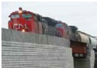
Handling Live Loads
