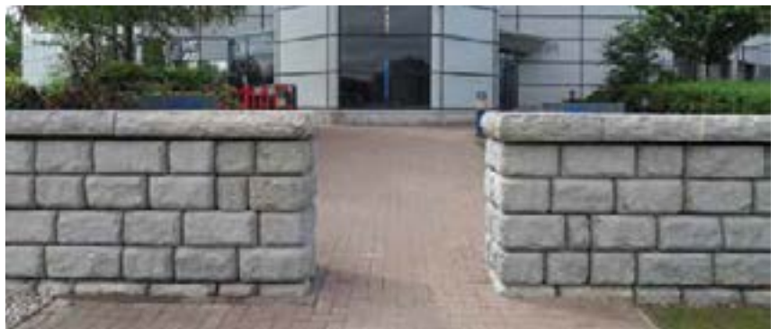
Build Barrier and Force Protection Walls
