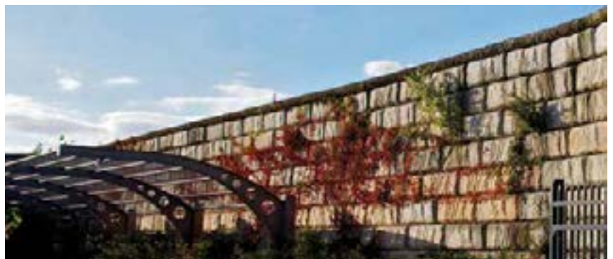
Finish Your Retaining Wall
